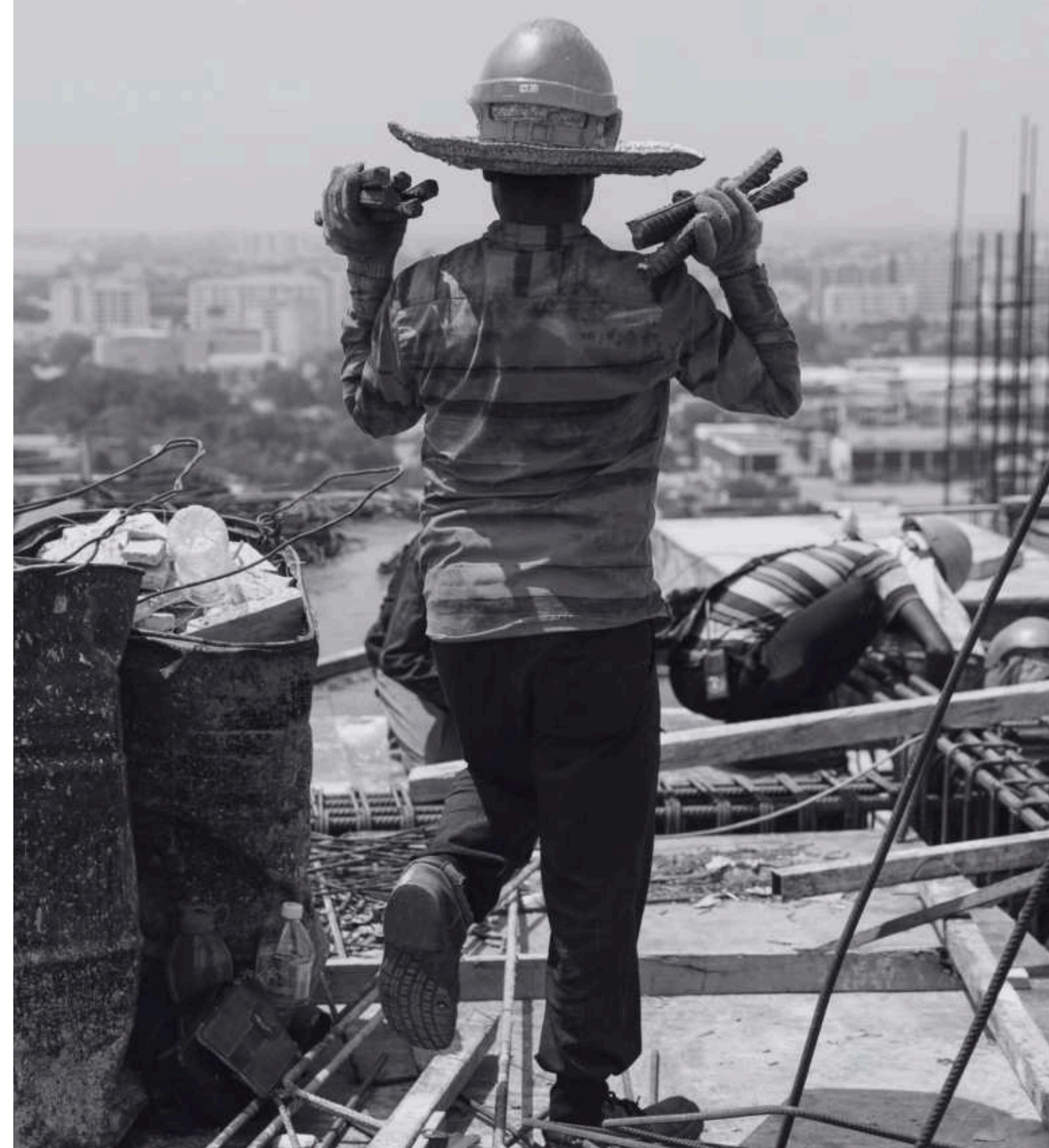
Rohingya workers employed on a construction site in Penang. Construction sites, which are numerous in Malaysia, are one of the few ways the Rohingya can earn a living in the informal economy, but some employers take advantage of their irregular legal status to deprive them of their full wages. (Penang, Malaysia, Apr 2019) | © Arnaud Finistre
